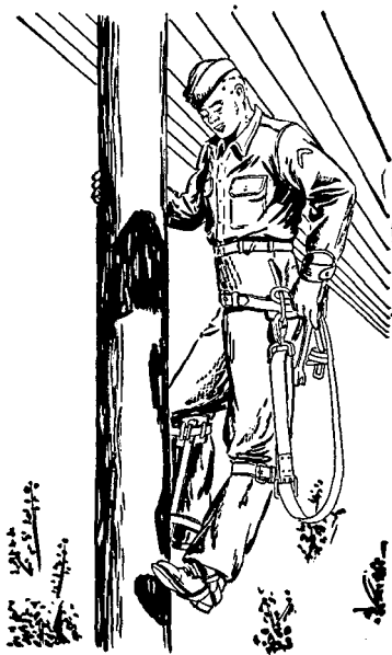
Figure 48. Unhooking safety strap.
