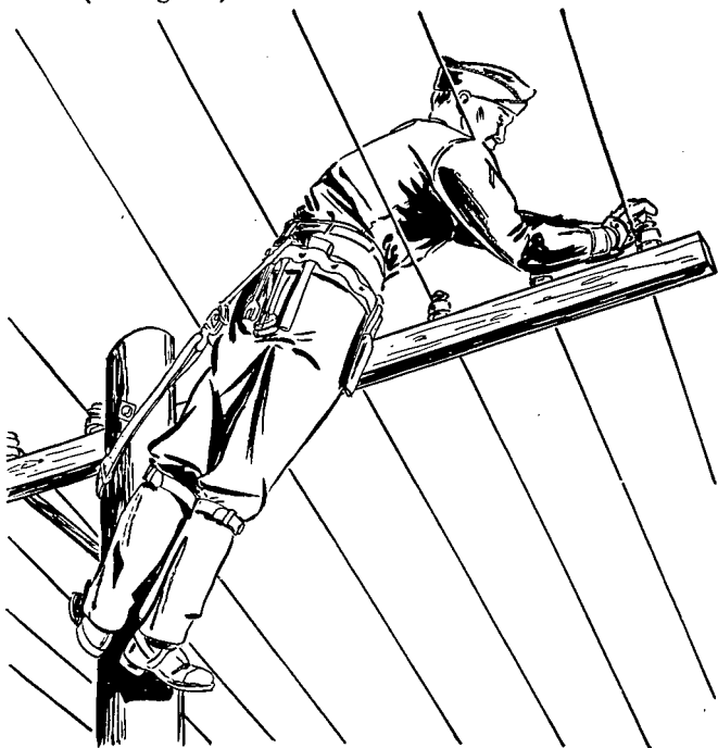
Figure 52. Working on outer wire of cross arm.
